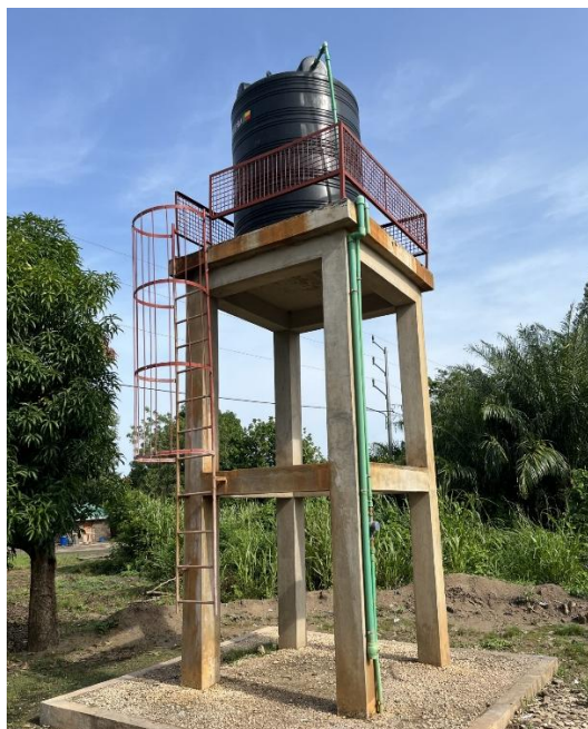
Photo 1: Water tower in Tohou
